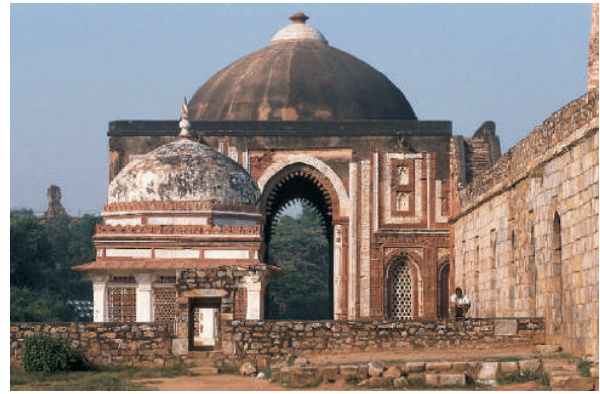
The Alai Darwaza erected in 1311 by Alauddin Khalji is one of the earliest buildings in India to employ the Islamic principle of arched construction
